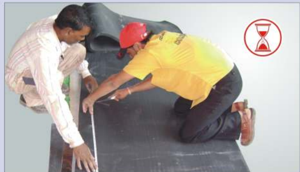
Manpower intensive work - Marking & Cutting
